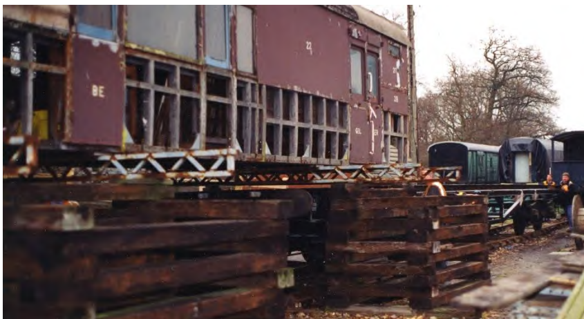
3687 coach body in the pump house siding at Horsted Keynes while its underframe is being carefully put back under it, 1996. Photo: John Arkell
