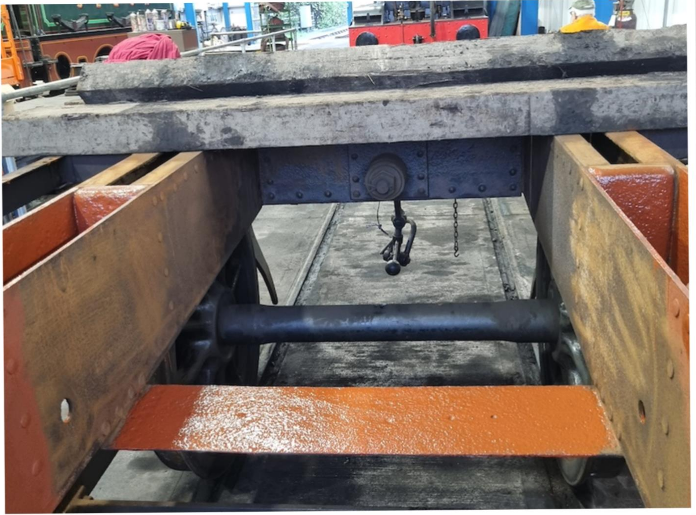
Above: Progress with cleaning and painting 541's inner tender frames. Photo: Steve Pilcher
