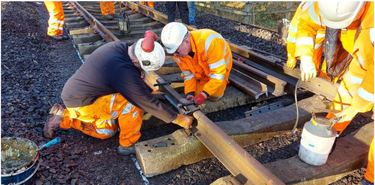
Plenty of grease on the plate bearing surfaces and on the bolt threads. Bolts done up with a Milwaukee impact driver but then finally tightened up with a hand spanner.
