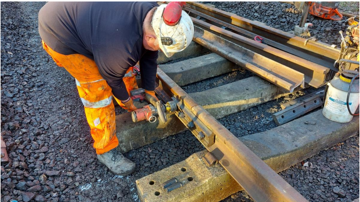
Plenty of grease on the plate bearing surfaces and on the bolt threads. Bolts done up with a Milwaukee impact driver but then finally tightened up with a hand spanner.
