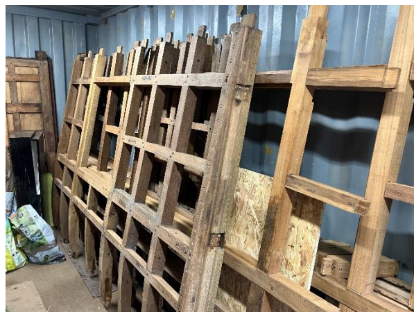
The growing stock of repaired frame sections in storage, pictured on 11 Jun 2025. The section at the front of the pile comprises pillars 22E-29E, being the section of the east side that forms the exterior wall of the pantry.
