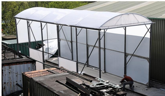
Covering the newly erected 40' long Poly-Shed
