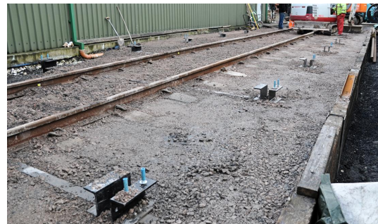
The new work area with track and shed anchors.
